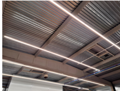
By switching from conventional fluorescent lighting to LED lighting, GC Europe saved 52% in energy use for lighting and reduced the time needed for maintenance.
