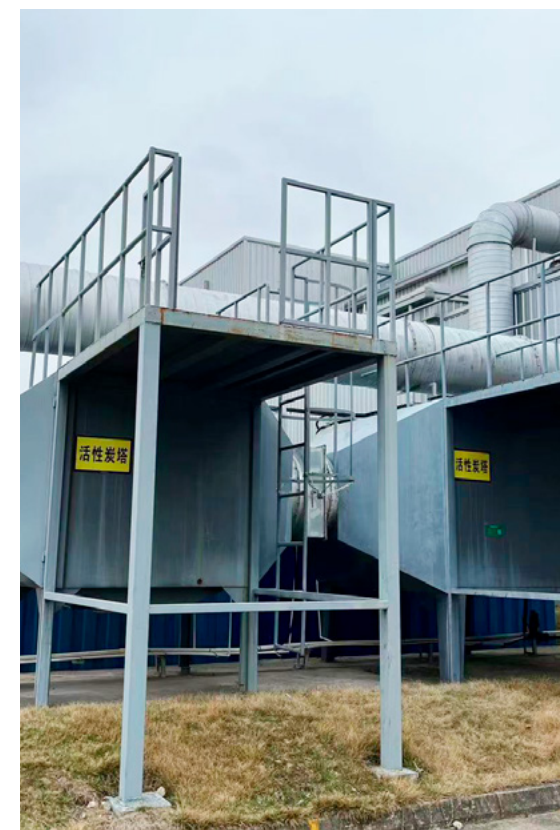
Double activated carbon facility at GC Suzhou
